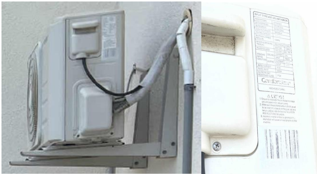
Figure 2: Split DX Air Conditioning System
